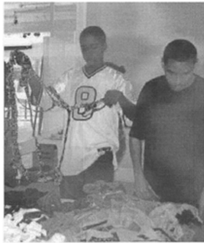
Wesley Frasier and James Barros examine seam "skeletons" prior to installation.
